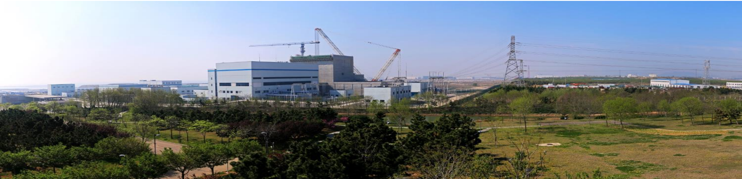
A View of the HTR-PM Site
