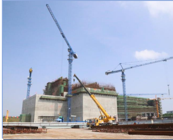
Civil work of nuclear island
