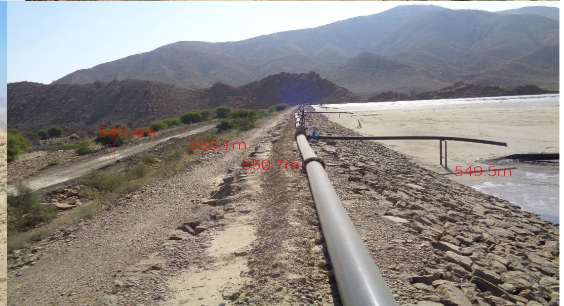
Tailings dam discharge facilities
