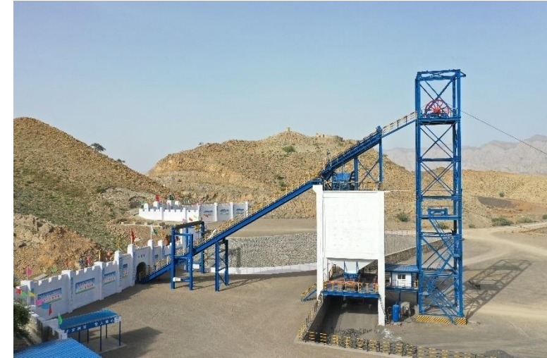
Inclined Shaft Operation Site
