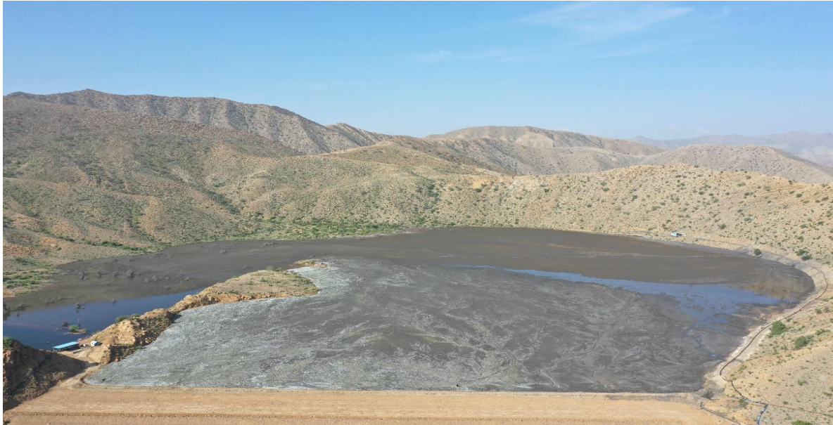
Full view of the tailings dam
