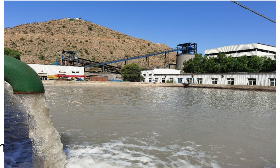
Industrial backwater sedimentation tanks
