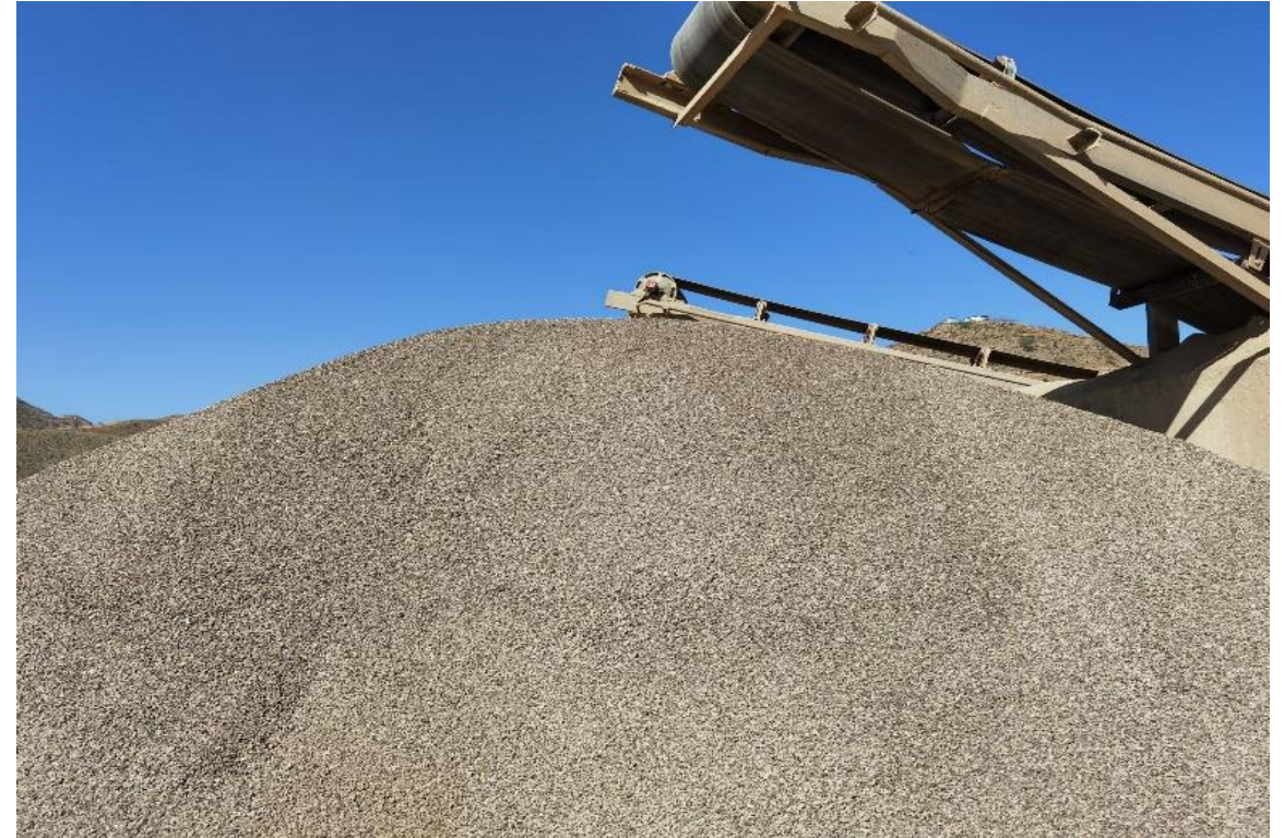
Crushing of waste rock to produce infill aggregates
