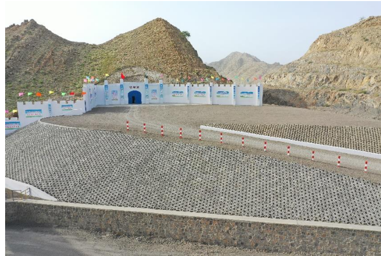
Ramp Work Site
