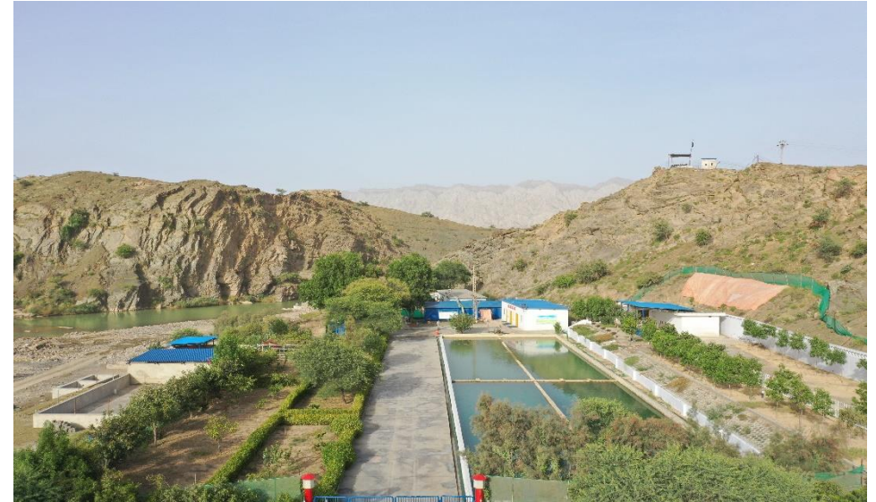
Rainwater and mine water sedimentation and purification ponds
