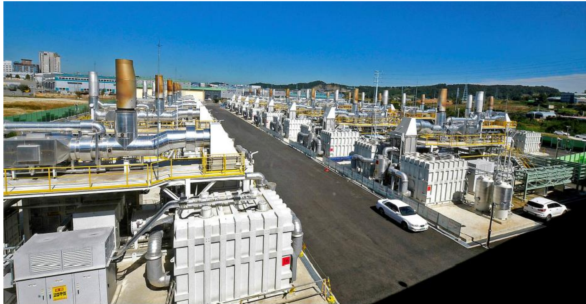
The world's largest fuel cell plant. 58.8 MW molten carbonate fuel cell park in Whasung City, Gyeonggi Province, South Korea (courtesy of FuelCell Energy Solutions)
