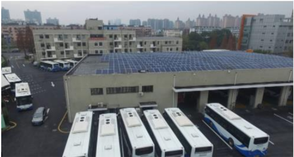
Fig.No.2 Shanghai city bus depot rooftop PV system [2]
